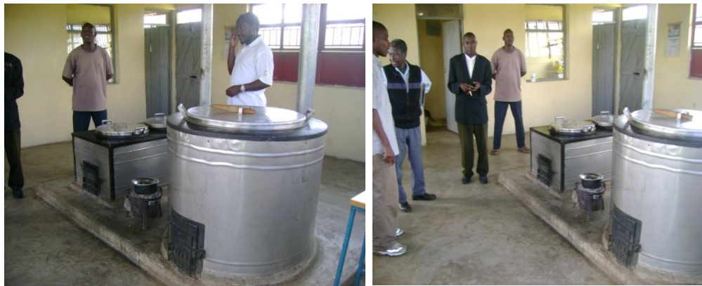
Highly Efficient Biomass Stove Set Up in a Private School (Bridgewater Girls Secondary School at Nakuru)
