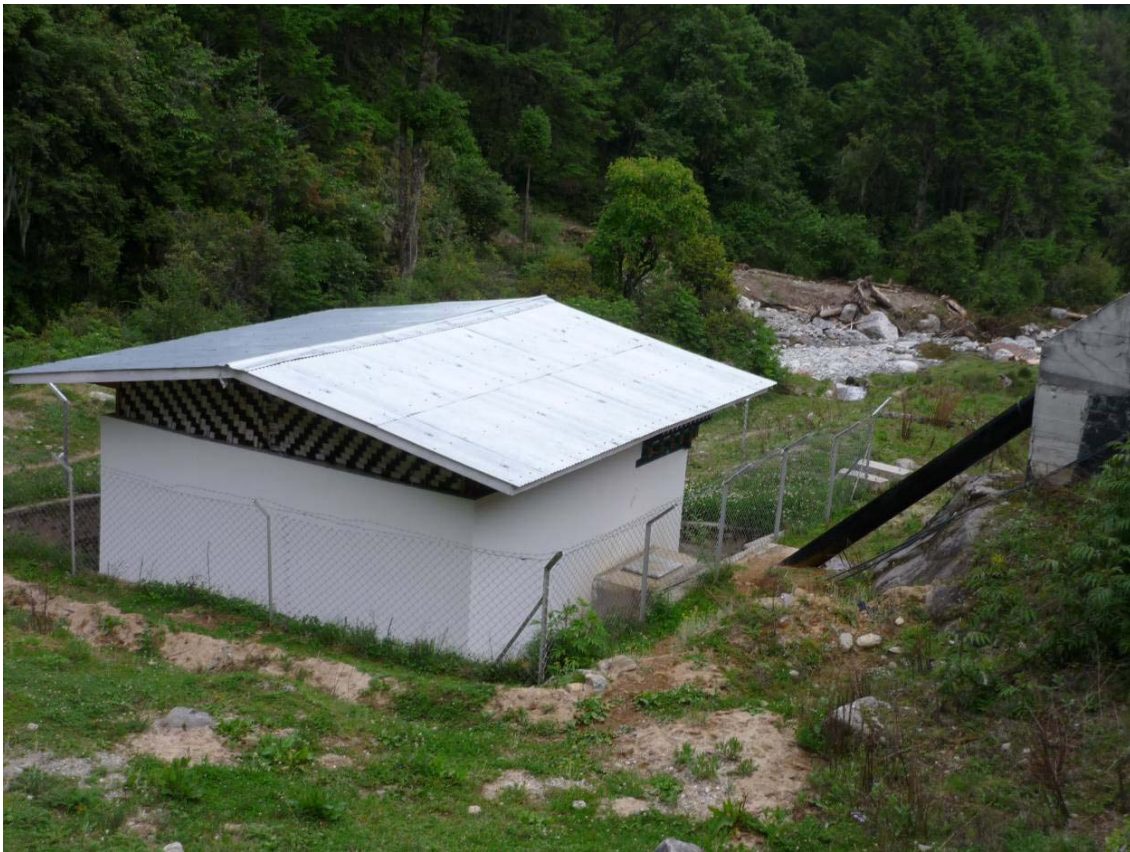
Sengor micro hydro power house and penstock with debris from recent flood in riverbed in background
