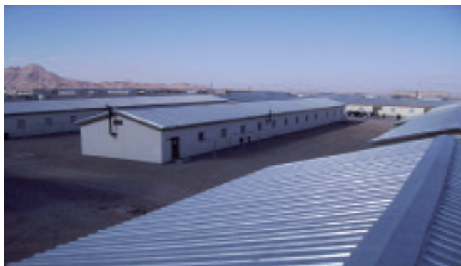
Photo 1. Herat – ANA dormitories
