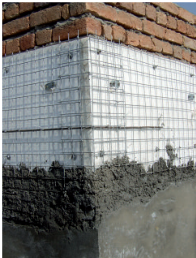
Photo 10 : External insulation (demo wall)
