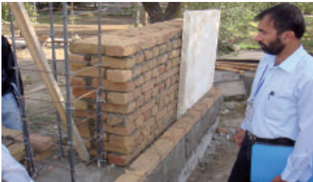
Photo 7. Double wall with polystyrene insulation
