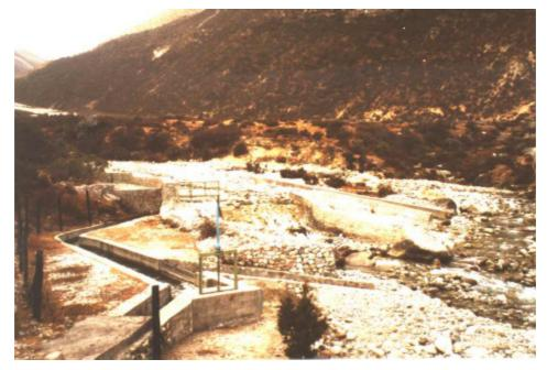
Figure 7: The intake area of the Namche SHP at Thame; in the foreground the desander
