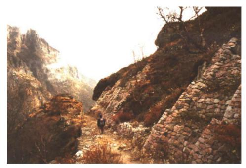
*Figure 9: Along the transversal course of the penstock, considerable slope stabilisation had to be implemented with high retention walls and shrub planting.*
