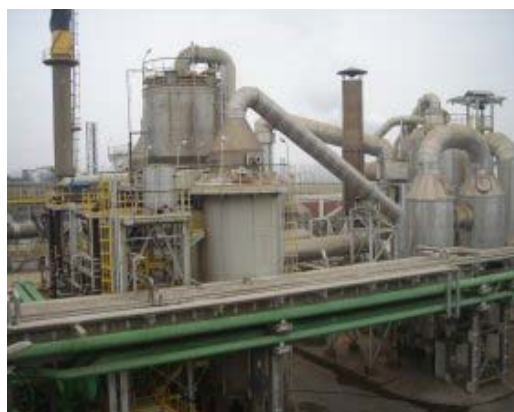
Renovated KCM Plant
