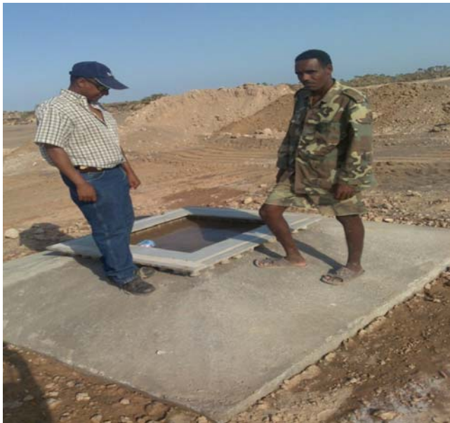
Photo: Completed foundation at the project site
