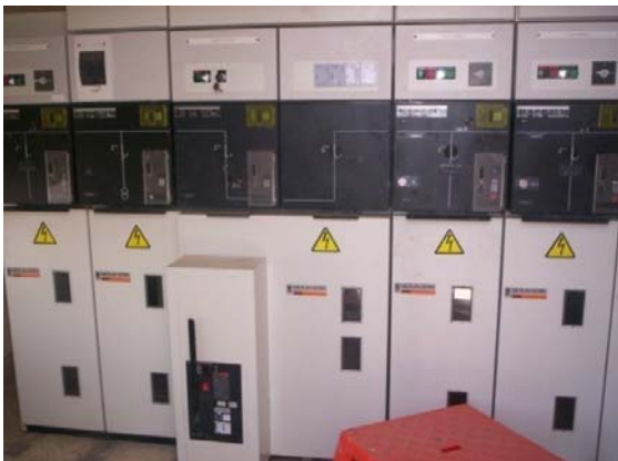
Photo: Switchgear to integrate Assab Wind Farm to the grid
